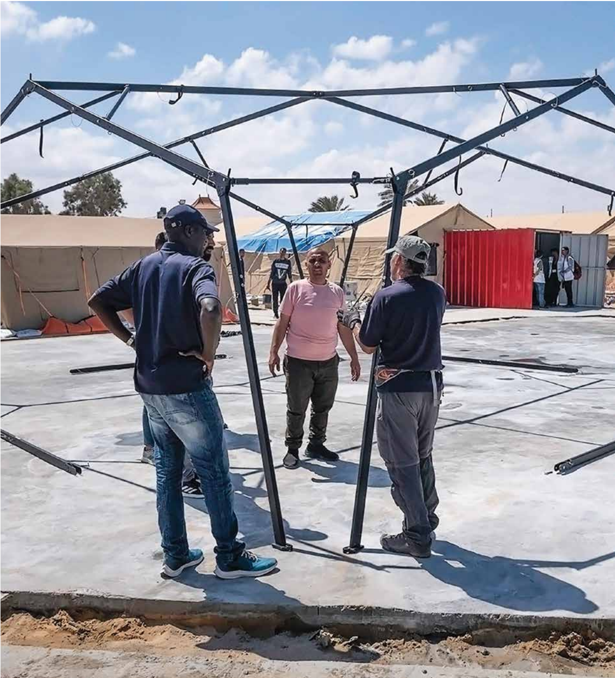
Operations support and logistics (OSL) staff setting up treatment structures, Gaza, Occupied Palestinian Territory, 2024. © UK-Med
